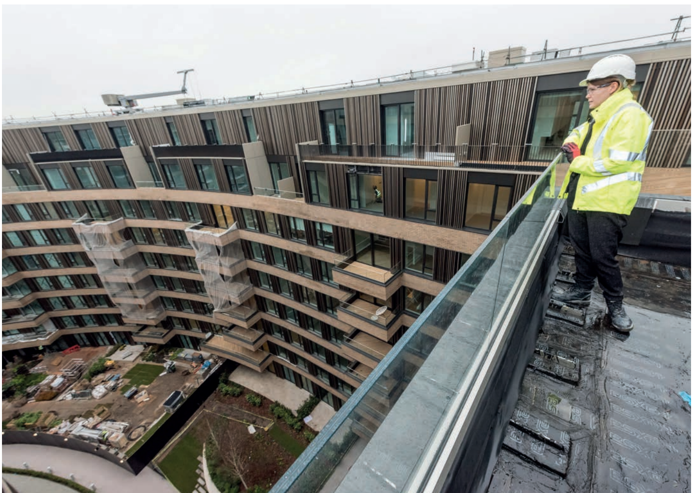
Engineer overlooks site © Arup
