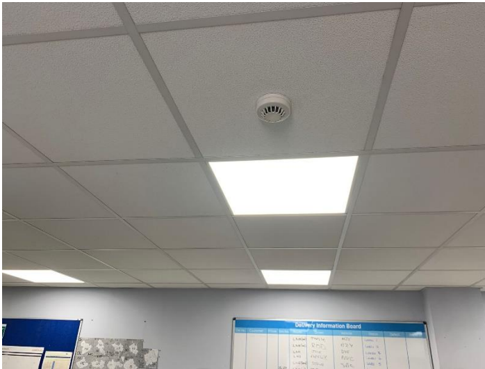
No mechanical air handling – extract or fresh air intake
